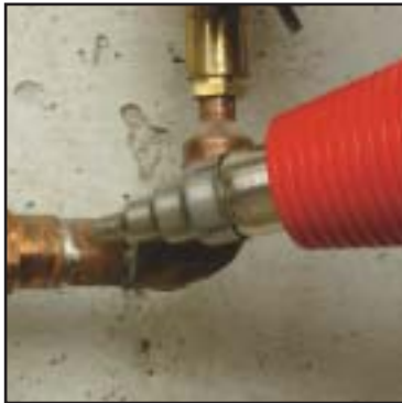
Solder Copper Pipe
